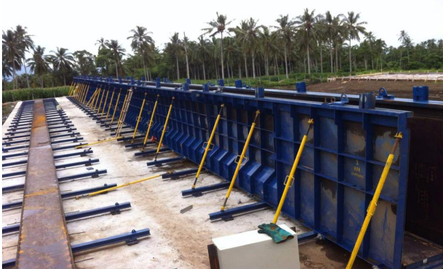
Fabricate and Install “Molding PCI GIRDER”
